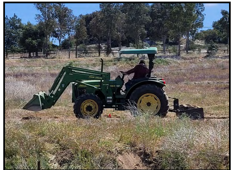
Rick Northcote grading the roadway for the mine train track.
