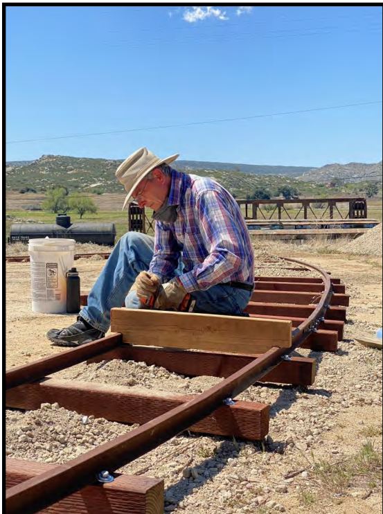
(Left) Tim Miller secures the rail to the wooden ties.
