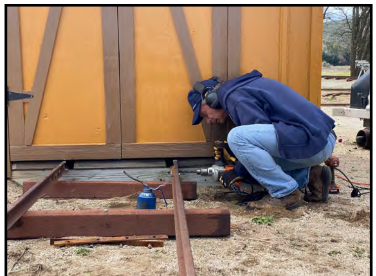
(Right) Steve Pohjola drills holes for a rail joint bar.
