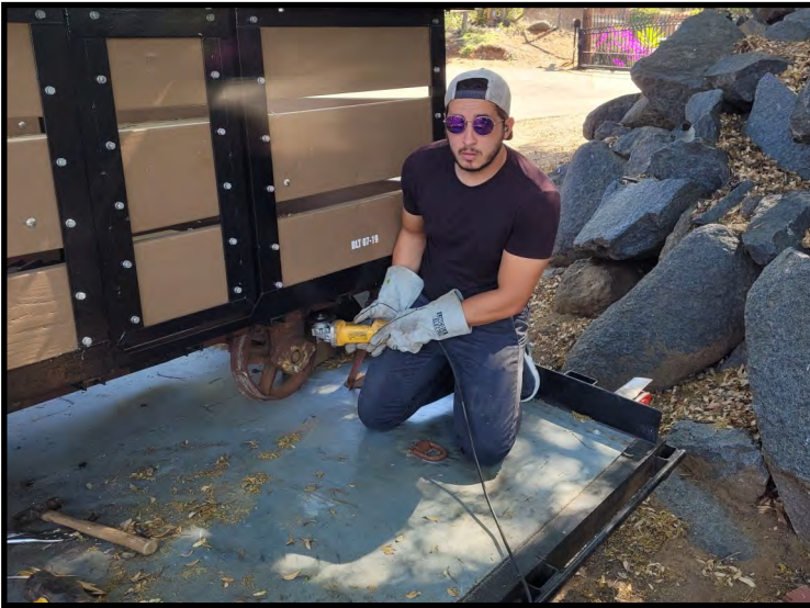
Diego Lundquist works to remove the old wheels under a mine train car to allow the installation of new roller bearing wheels.
