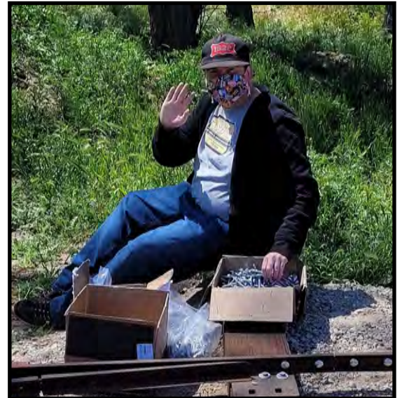
BG Miller working hard to put together washers with lag bolts used to secure the rail to the ties of the mine train.
