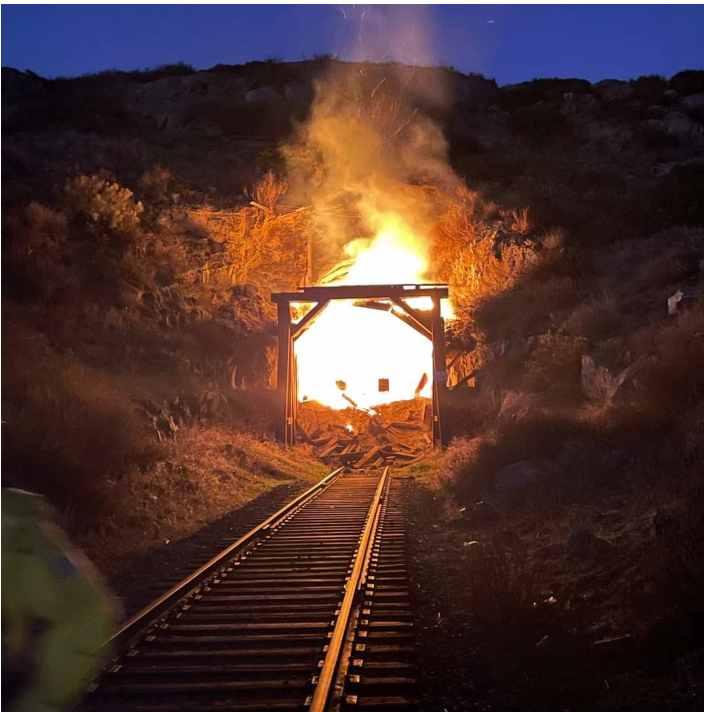
Looking at tunnel 4 western (southern) portal on fire from the Mexican side. The border is just inside the tunnel. Photo from internet
