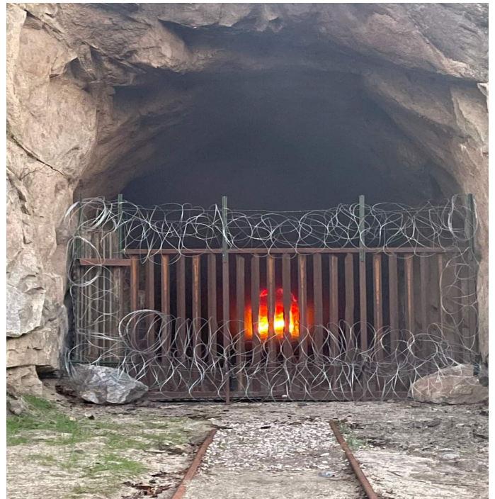
Looking at tunnel 4 from the eastern (northern) portal at the fire from the Mexican side. The gate is considered temporary. Photo from internet
