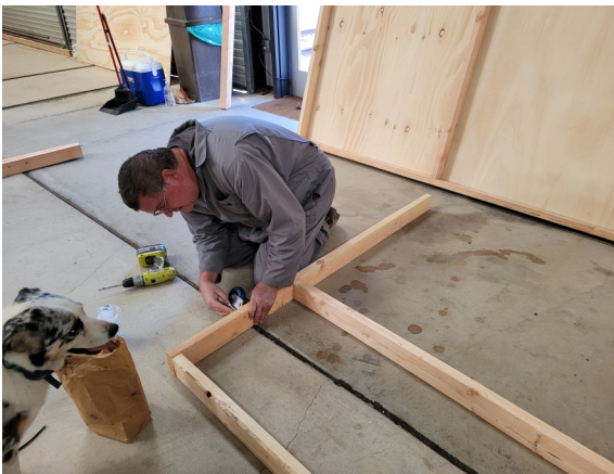
Jim Lundquist constructing walls Photo by Dawn Lundquist 1/12/22
