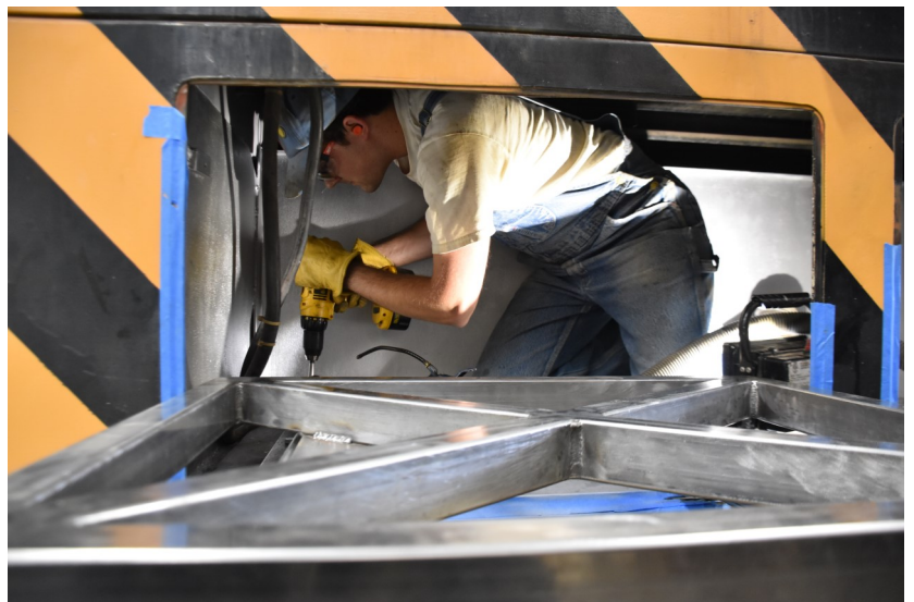
Stephen Hager prepping battery box for installation of trays
