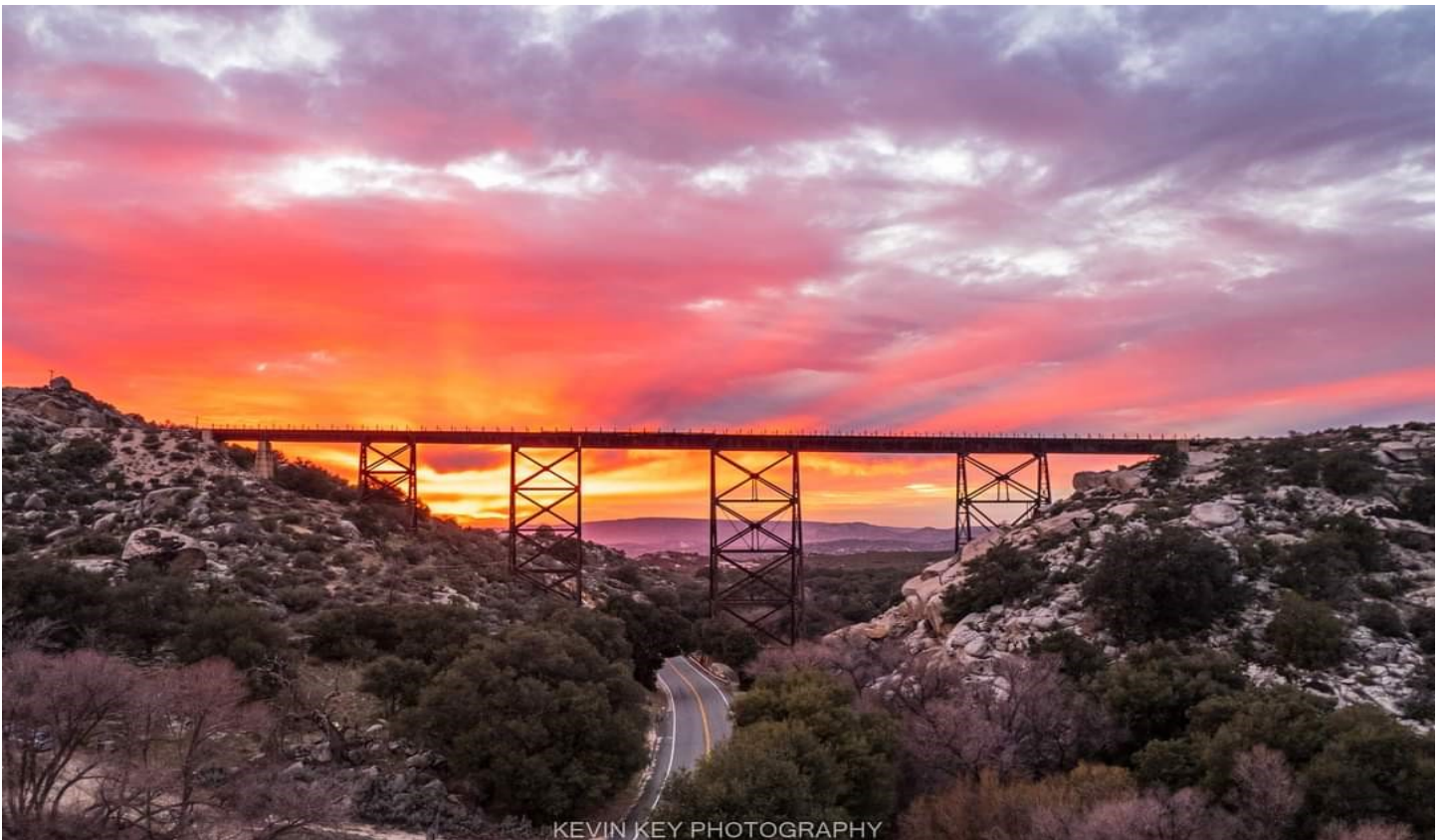
Sunset behind the Campo Creek Viaduct in the east end of the Campo Valley. The 1916 SD&A bridge is located at Mile Post 77.27, which is 12 miles east of the Campo Depot. Simply a stunning photograph.
