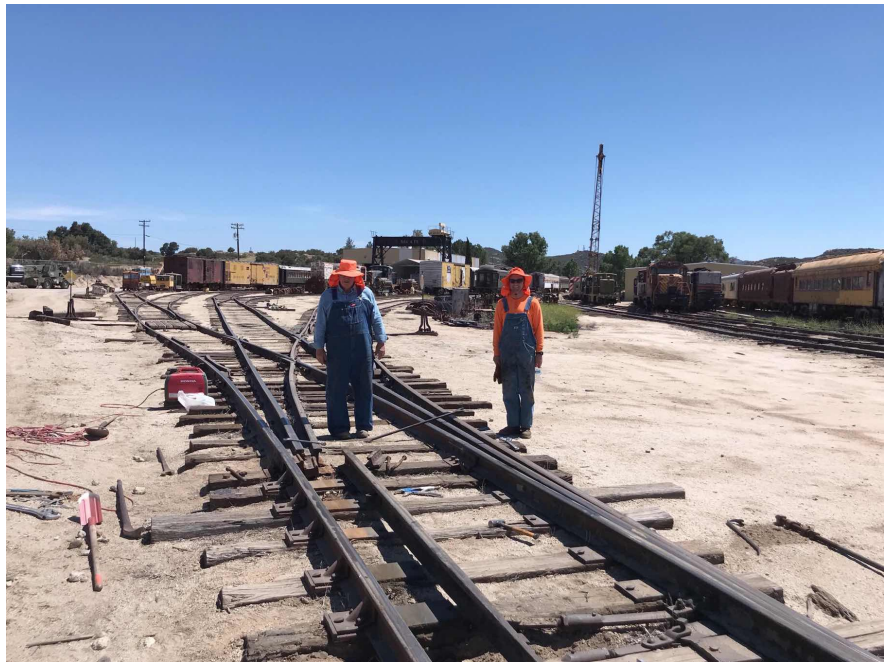
Roadmaster Glen Rogers and Track Foreman James Caestecker pose with the Santa Fe Triple Switch with the switch points disassembled. Photo by Frank Najera.
