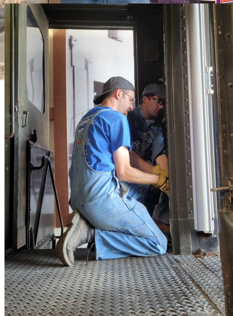
(right) Martin Caestecker and Stephen Hager continue the effort of installing new hand brakes.
