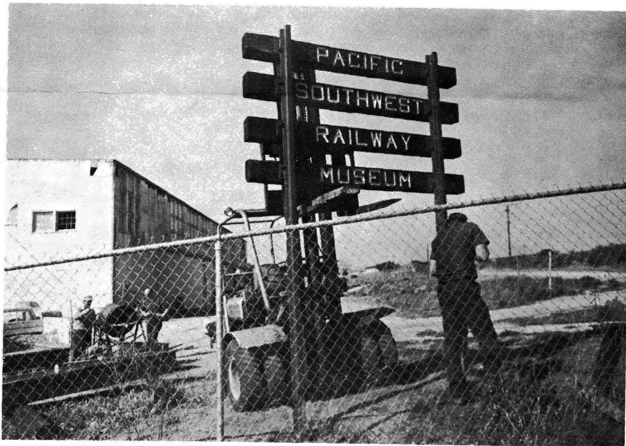
Museum Executive Director Jim Lundquist is shown here tamping concrete around the posts of our new sign that was built by Harry Doering. Harry and Roger Garrett are running the cement mixer in the rear left. (L. Rose photo)
