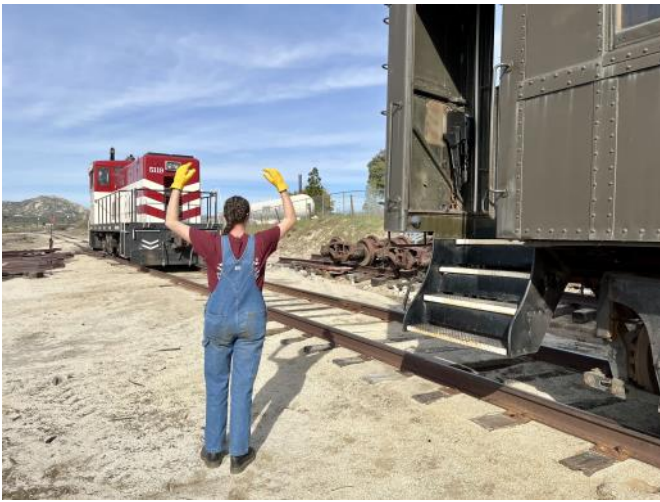
Directing the Engineer to come into a joint.
