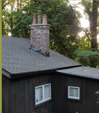
Wisteria with New Roof
