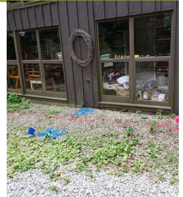
Top House is now anchored to Bedrock
