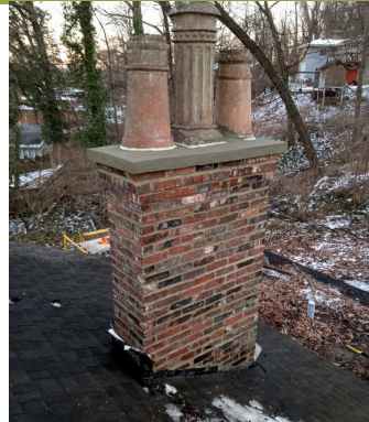
New Chimney on Wisteria
