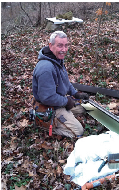
Ron Washburn at work on the gutters.
