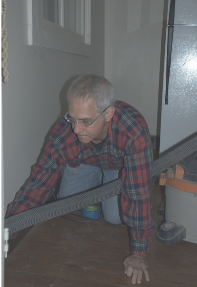
Kevin Karl prepares the kitchen for painting
