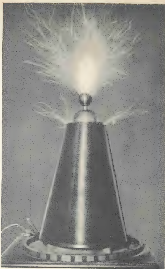
Dr. Strong's Million Volt Coil in action, giving a tree-like flaming discharge nearly four feet high
