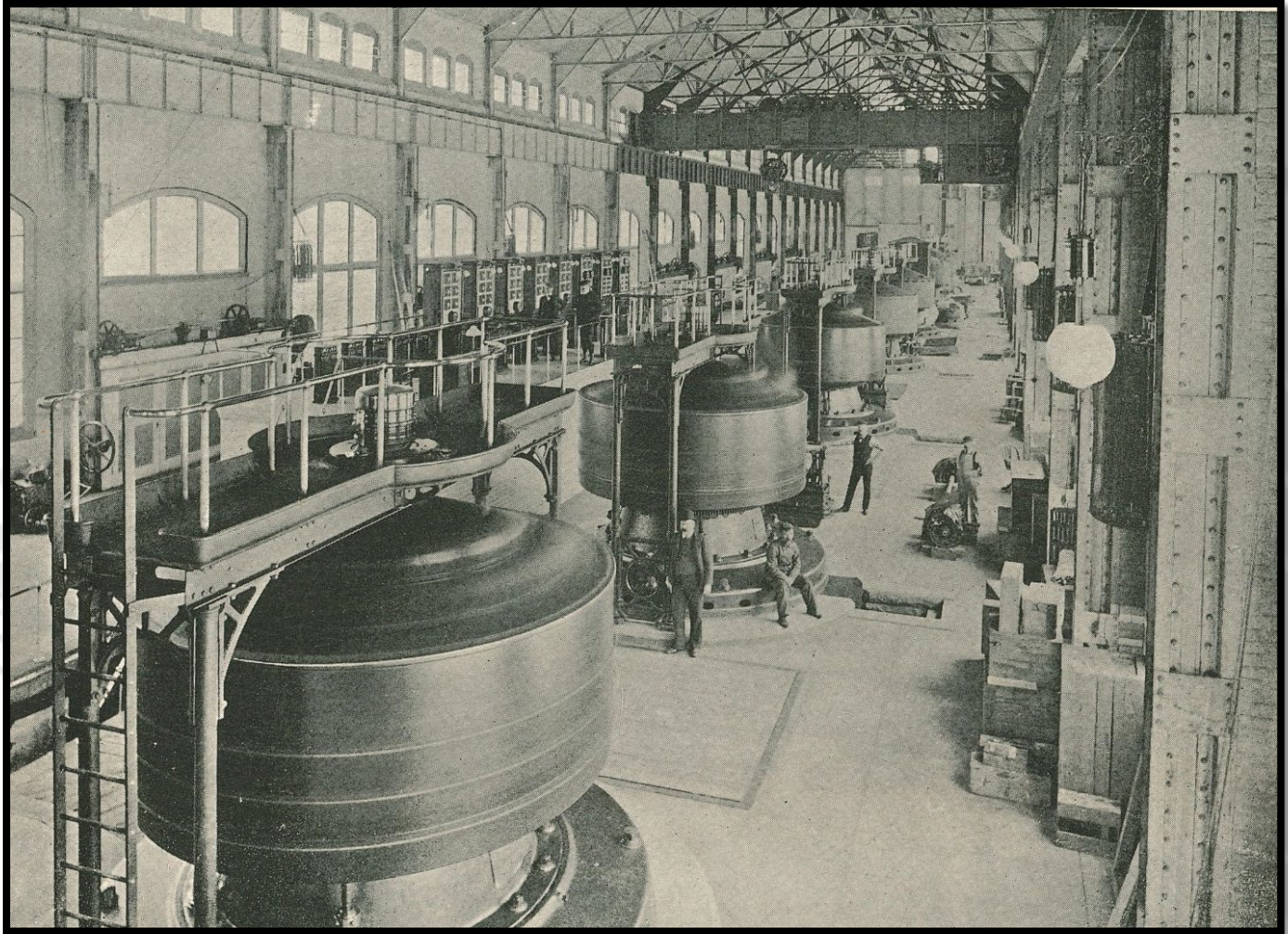
Interior view of power house showing the gigantic generators whose power is utilized by numerous railroads and manufacturing plants. Niagara Falls, L. H. Nelson Co., 1904, Published for S. H. Knox & Company
