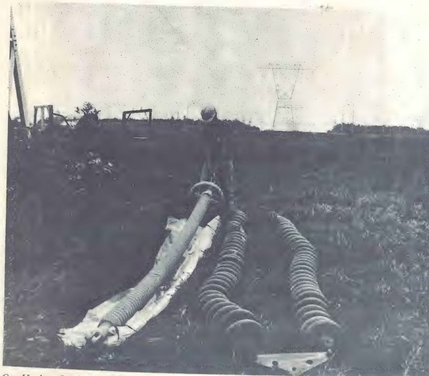
On Hydro-Quebec's 735-kv transmission lines a single element synthetic insulator weighing only 32 kilograms may replace two-string porcelain insulators (right) weighing 548 kilograms.
