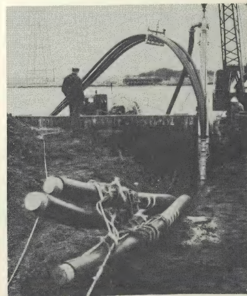
HYDRO-JETTER UNIT: 1-water-pressure hose; 2-injector; 3-plastic conduit to be embedded in river bottom; 4-winch line; 5-free-running conduit coils
