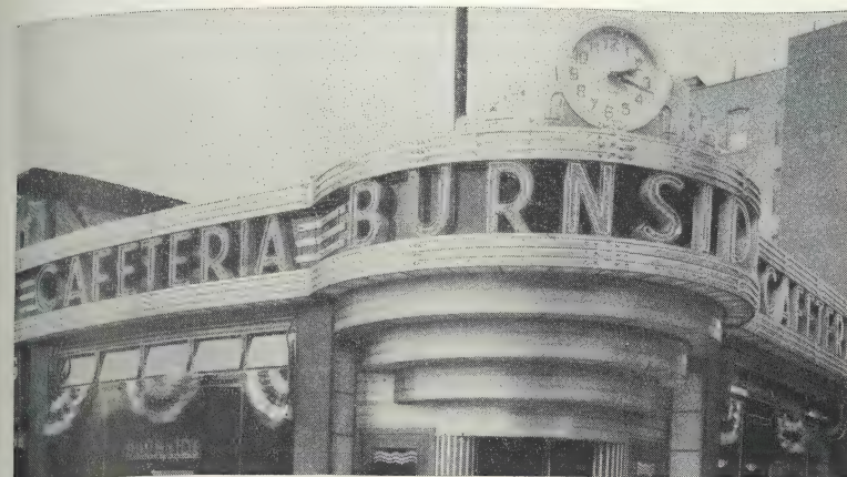
FIG. 29.—Outline skeleton sign applied as a triple-tube unit.
