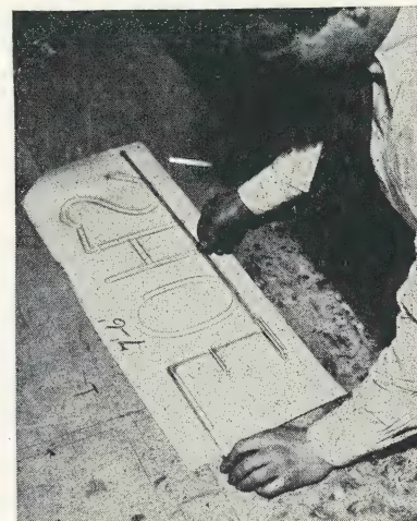
FIG. 54.—Matching letter to asbestos layout.
