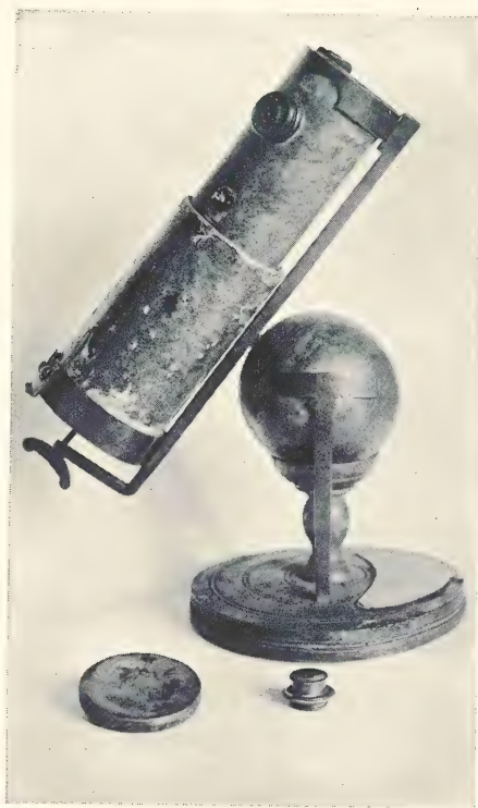
A. The old inscription on the base runs:—THE FIRST REFLECTING TELESCOPE INVENTED BY SIR ISAAC NEWTON AND MADE WITH HIS OWN HANDS IN THE YEAR 1671. By permission of the Officers of the Royal Society. Height about 18in. (p.107)
