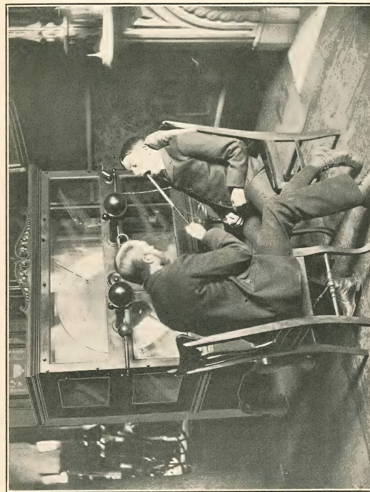
PLATE III.—Administration of the High-Frequency Current with the Glass Electrode to the Fauces. The Electrode Connected by a Cord to the Negative Side of the Machine, Positive Side Grounded, and a Short Spark Discharging at the Spark-Gap.
