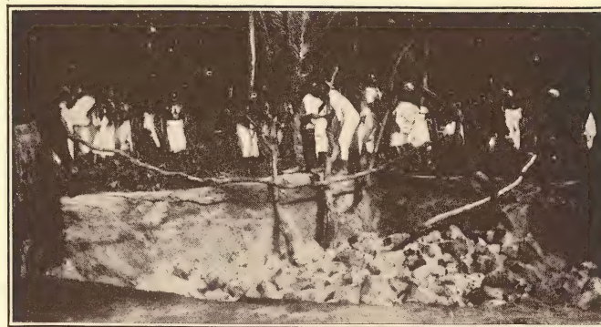
LOWERING THE GREEN LEVELING VINE INTO PLACE
