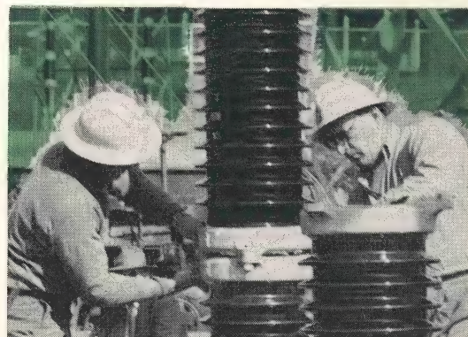
5 Second flange connection is made with men still standing on the ground.
