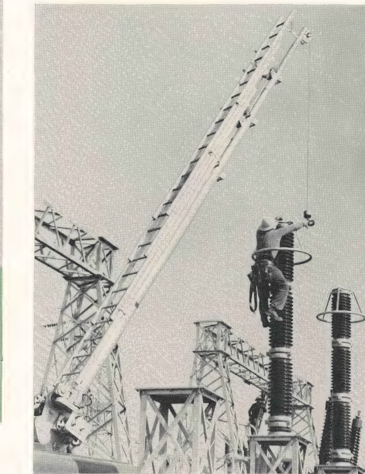
10 Base mounting bolts are installed.
