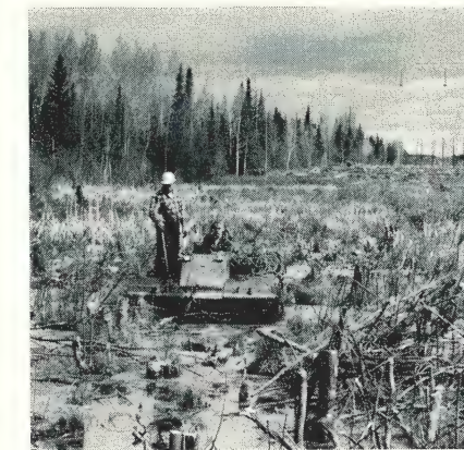
The first 100 miles south of Pinard Transformer Station crossed flat terrain covered with muskeg. Here, one of the special "muskeg buggies" crosses a section of heavily forested muskeg terrain.
