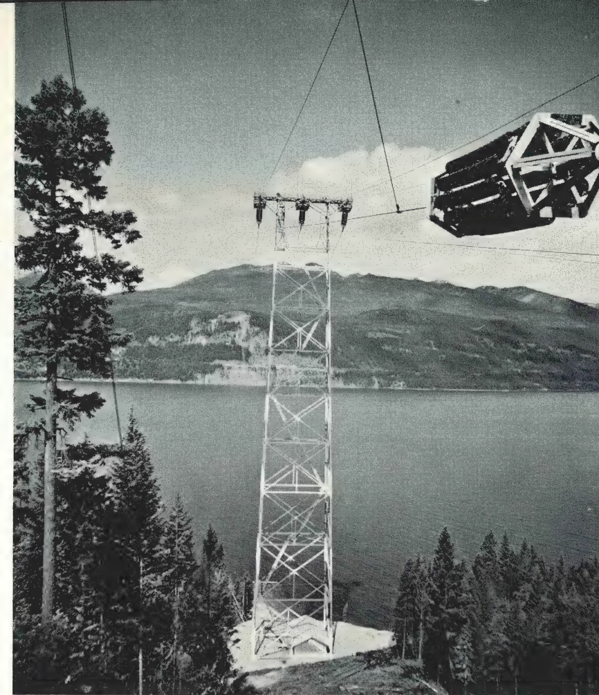
Figure 1 -- "Whiffletree" principle of multiple-string deadend that multiplies by 12 the strength rating of insulators used. In practice, this arrangement forms a hexagonal cylinder with points (A) joined. Load is divided and equally distributed on insulator strings.
