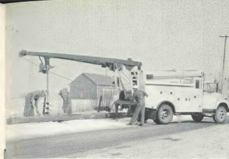
Series 6800 Derrick has extra cylinders for extra power in the low ranges. Here, with power feed attachment, it forces digger into tough ground. All equipment is Holan.
