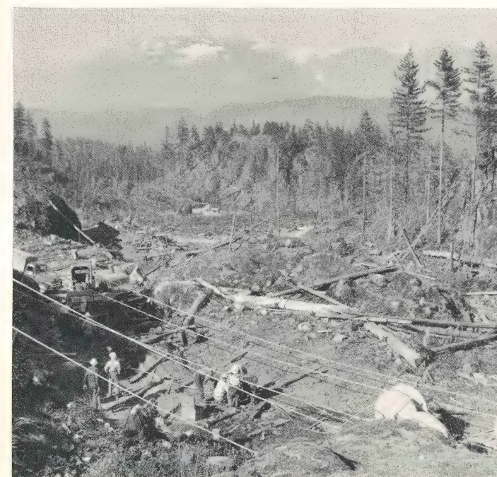
Stringing Rosedale, Creekside, Bridge River line through rough country near Lillooet Lake. Care was needed with conductor under tension to keep conductor off ground and rocks.
