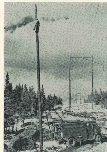
7. Spacer being installed on two-conductor bundle phase. Two types of spacers were used. One has a helical steel spring between clamping members. The other has an aluminum tube spacer.
