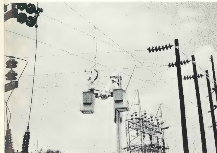
Three phases of a 69-kv cross bus being connected with permanent jumpers. Holan elbow safely puts crewmen within arm's reach of the job, relieves undue tension and eases problem of fatigue.
