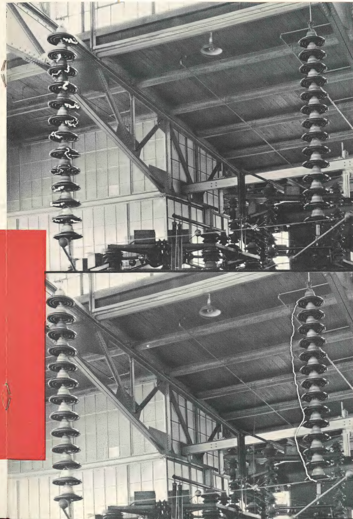
Here an overvoltage sufficient to cause a two microsecond flashover was applied. The string having the shorter cascade striking distance flashed over.
