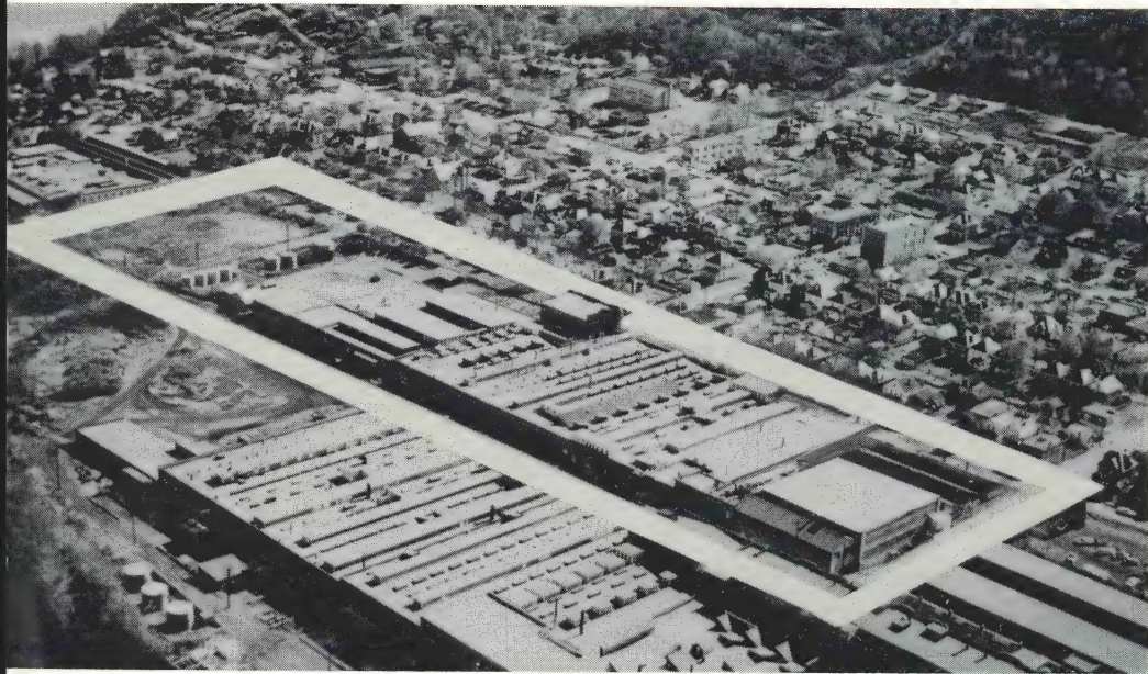
Aerial view of the 356,000-square-foot plant which will be converted as rapidly as possible into expanded manufacture of O-B insulators. Well over a year of construction and organization have been by-passed with the acquisition of this large ceramic plant.
