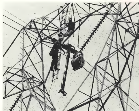
The linemen raise and guide the lifting yoke into position prior to removing the conductor load from the stringing blocks. Eighteen, 15,000-pounds insulators support each leg of the V-string.
