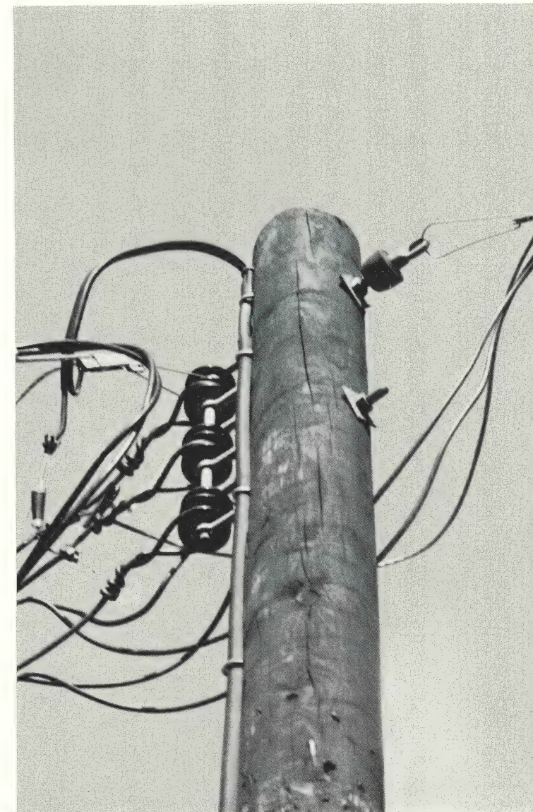
Here's a close-up of a Dirigo installation — note the Dirigo threaded on to the rack bolt. One utility's crews save 15 to 30 minutes in construction of this simple service drop.
