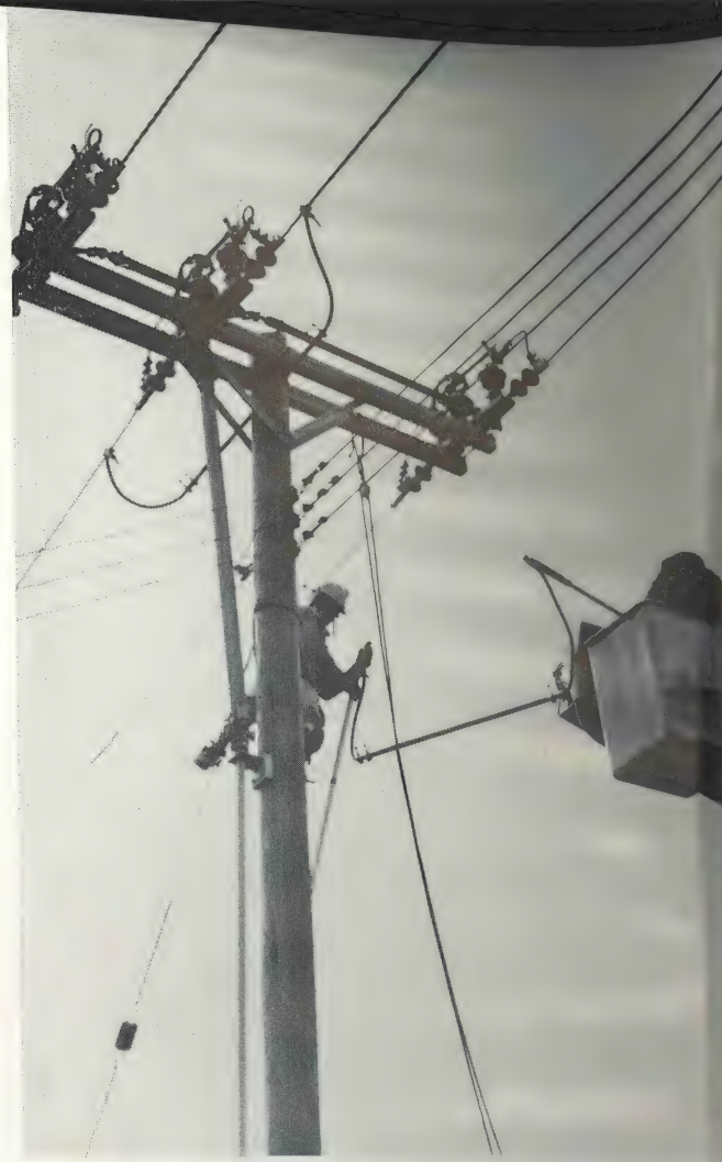
Linemen install by-pass jumpers, putting burned connectors out of service until permanent repairs can be made.
