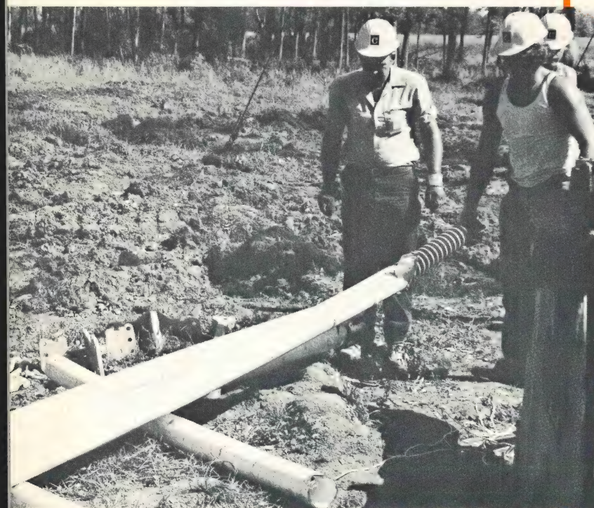
Unpacking a Hi*Lite insulator for a 500-kV line. The complete one-piece insulator has a weight of less than 50 pounds. Its porcelain equivalent would weigh 465 pounds and come in five separate shipping crates weighing 93 pounds each.
