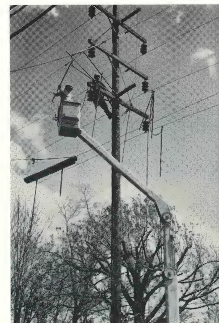
Working together, the man on the pole and the one in the 89's bucket installed the top phase of the energized 23.5-kv circuit. Then, the lineman in the 89 finished clipping in the lower two phases, assisted by the man on the pole.
