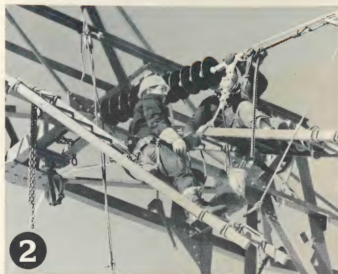
2 With insulators and clamp under tension, slack conductor is formed into clamp.
