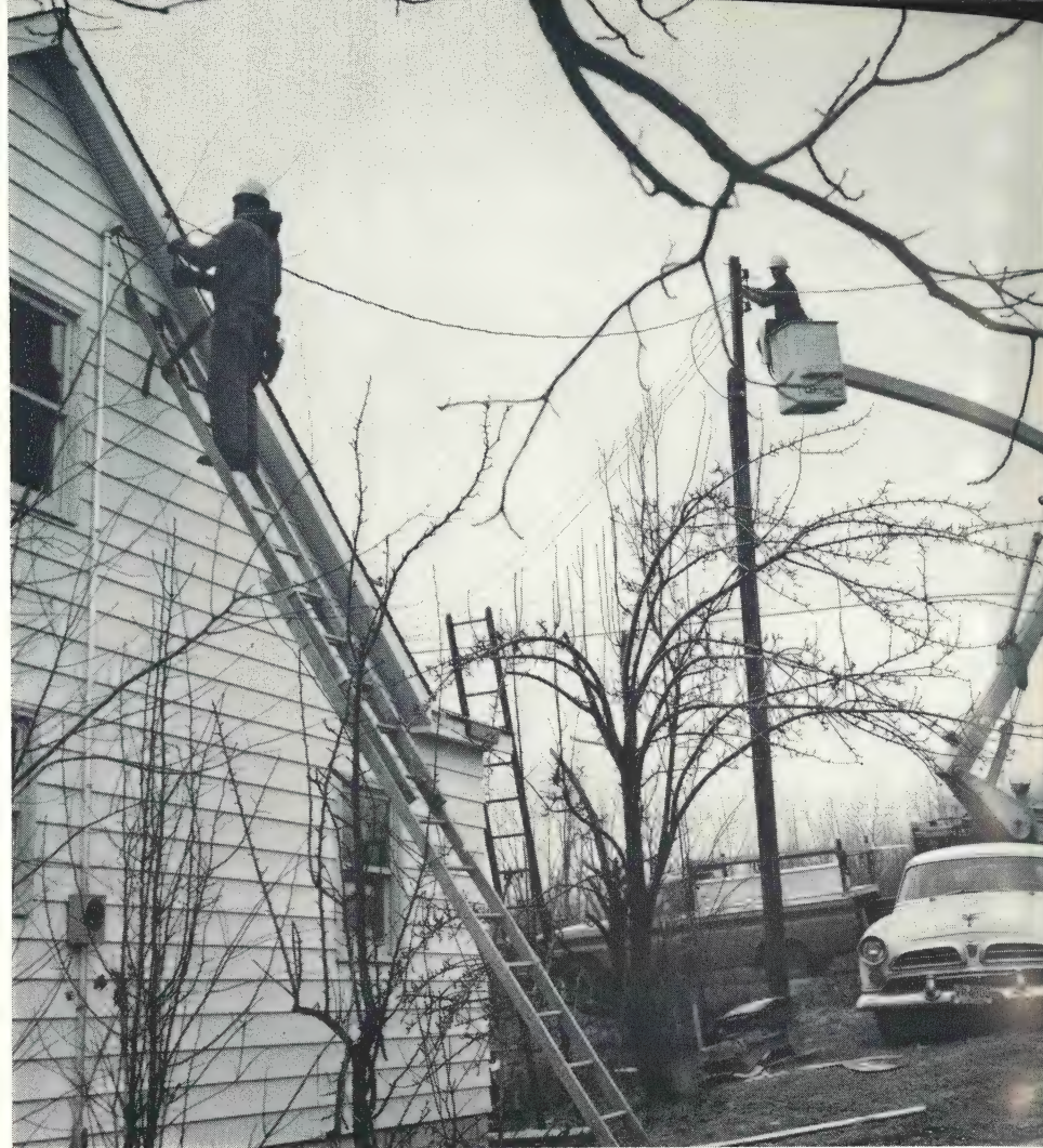
Maneuverable aerial elbow speeds installation of electrical service at a new residence.
