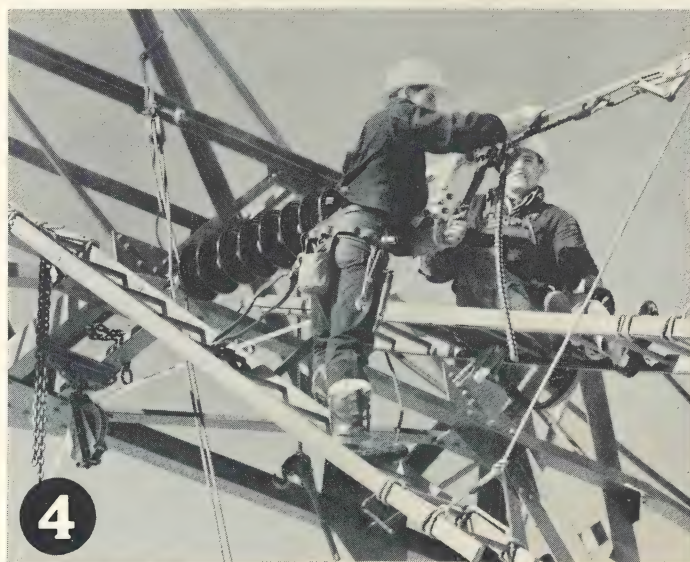
4 Tension is transferred to conductor when jack-hoist is removed.
