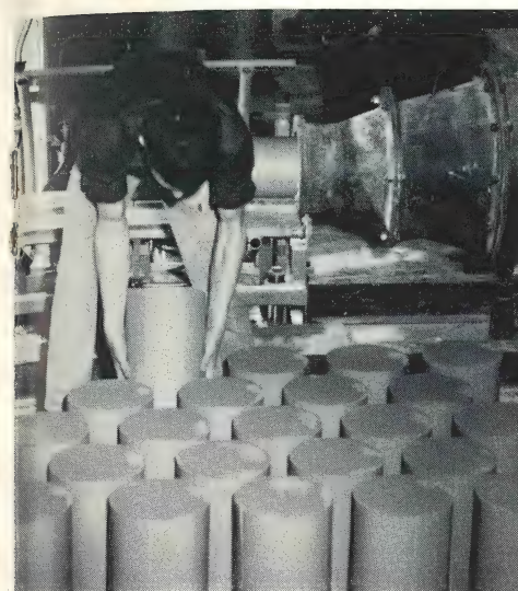
Newly extruded clay blanks stacked on pallet for transport to drying area.
