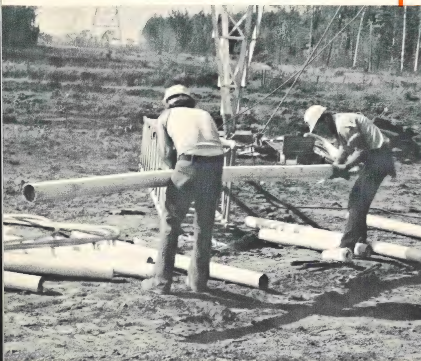
Unpacking a Hi*Lite insulator for a 500-kV line. The complete one-piece insulator has a weight of less than 50 pounds. Its porcelain equivalent would weigh 465 pounds and come in five separate shipping crates weighing 93 pounds each.
