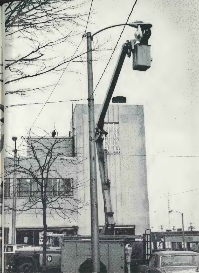
Fast-moving aerial bucket cuts time needed to replace lamps and photocells in city streetlights.
