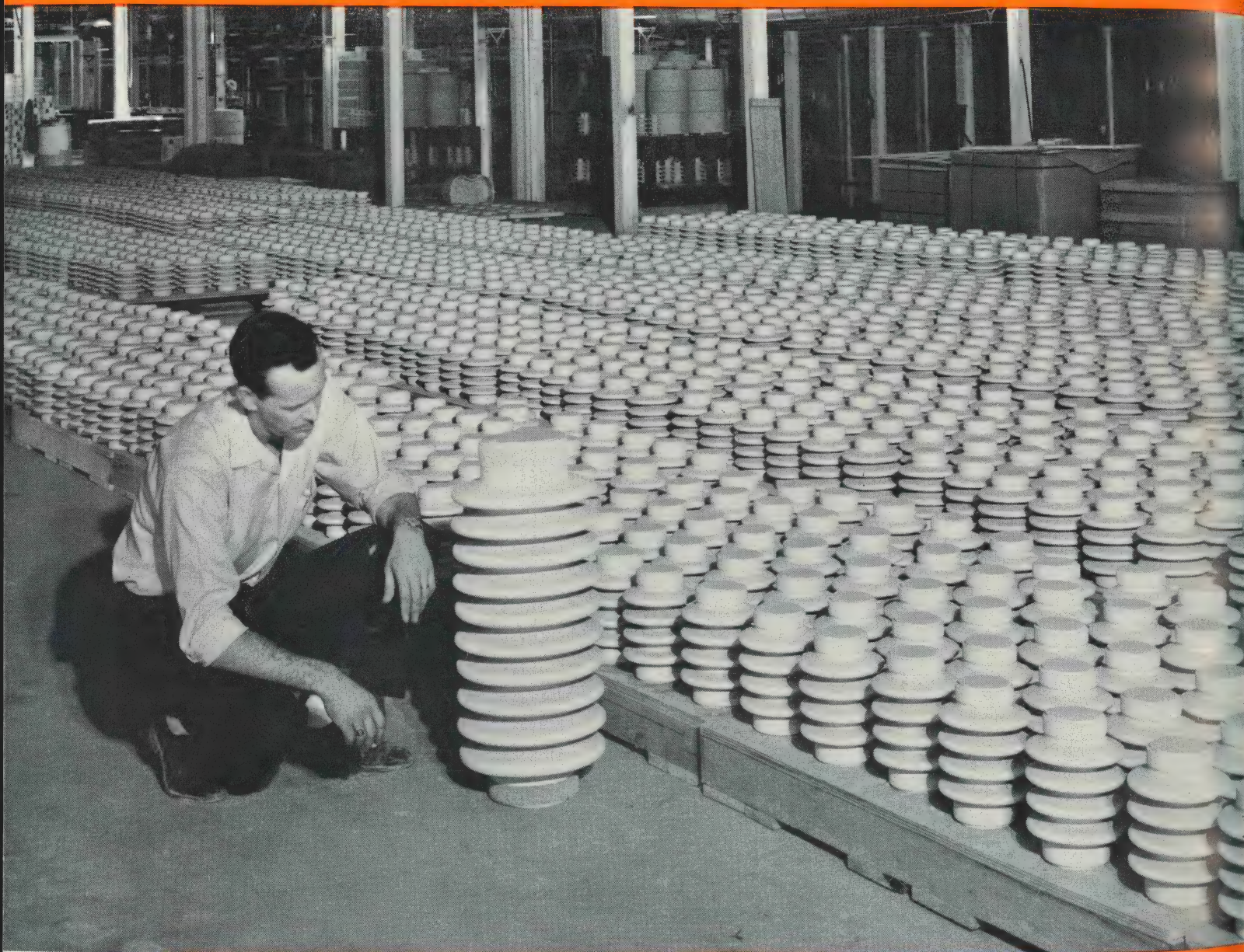
After forming and drying, post insulators are held in storage awaiting final finishing and glazing operations preparatory to firing through the tunnel kiln. This picture is indicative of Newell's present production of posts.
