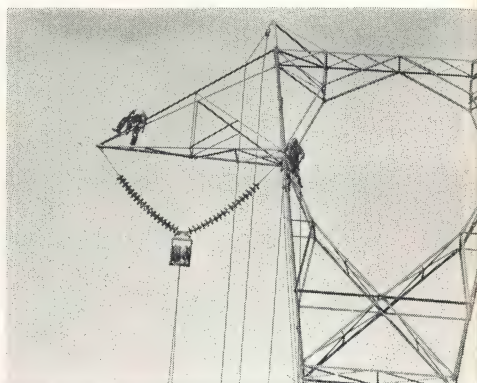
With the insulator-hardware installed in the left phase, the linemen carry their hand lines across the crossarm to prepare for receiving the next assembly.
