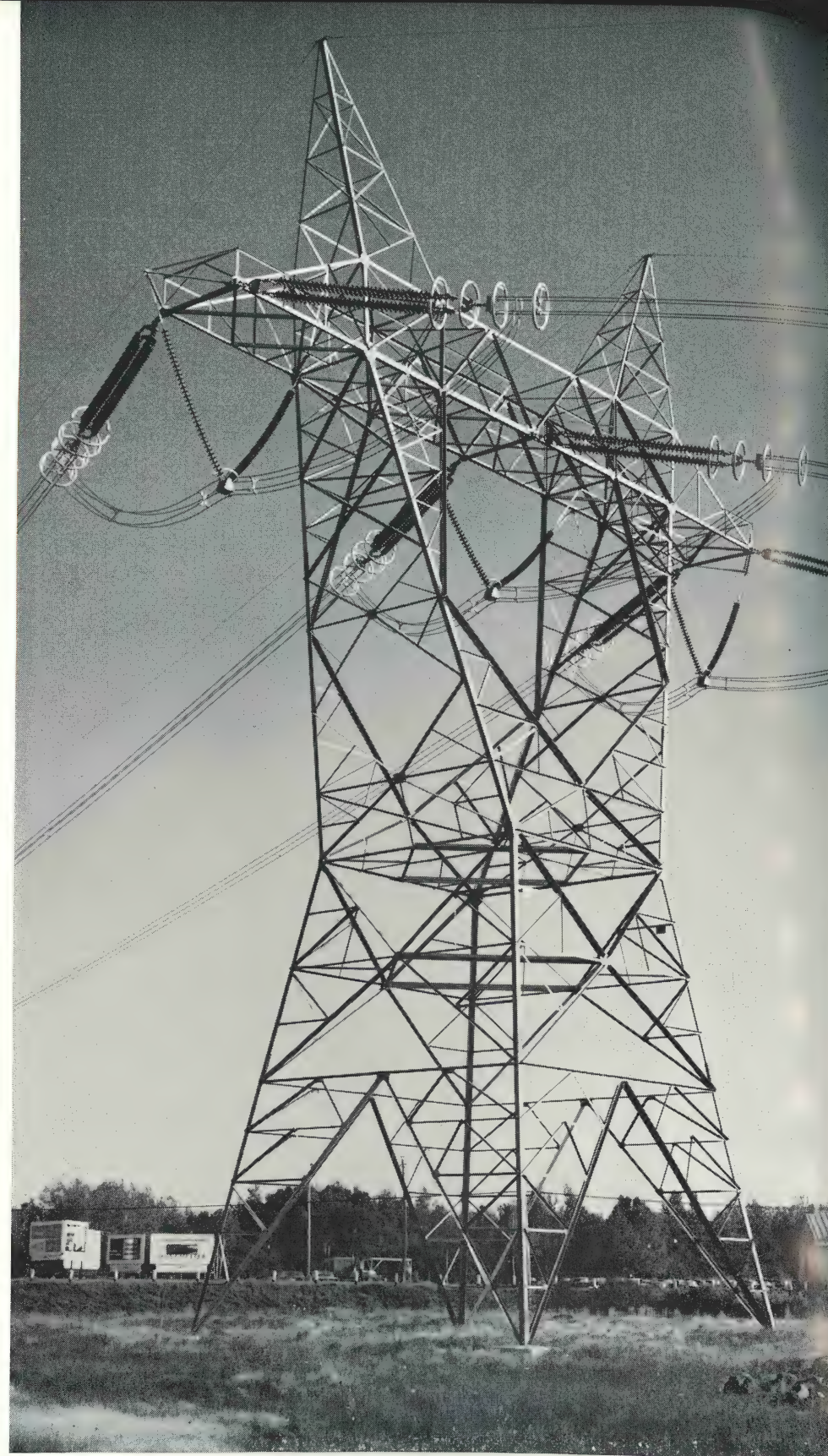
Type of strain tower used by Hydro-Quebec for angles of 15 to 30 degrees. This tower follows the practice applied throughout the line of 50-foot phase spacing and anchorage of conductors 110 feet above ground. The structure is un-guyed.
