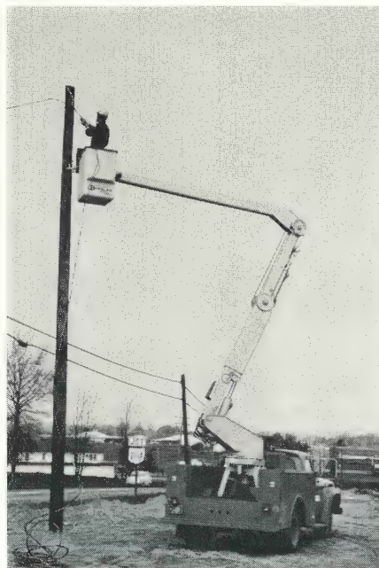
While work proceeded on the pole setting, the Bronco 89 went across town to install a new service drop. Without outrigger jacks to set, a lineman gets up to the pole fast in the 89.
