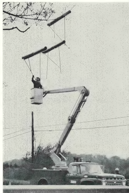
To provide clearance for setting the new 65-foot pole, one lineman used the new Bronco 89-36-3 to attach roller link sticks at midspan and float the energized 23.5-kv circuit away.
