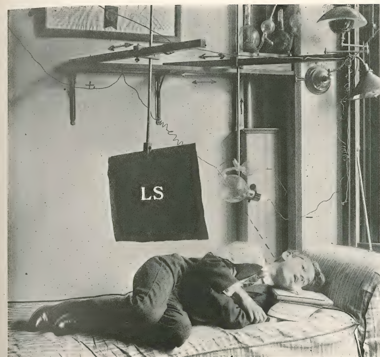
FIG. 200.—EXTRA-ORAL METHOD IN DENTAL SKIAGRAPHY.—LS, lead screen for the protection of the operator. The arrows indicate the variable positions to which the author's tube-holder may be shifted. The illustration depicts the sensitive plate placed upon a book and the lad's left (suspected side) cheek resting on the plate, the dotted line shows the path of the rays.
