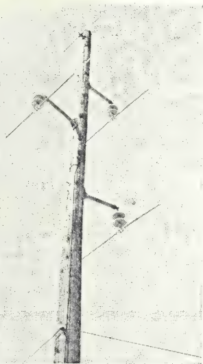
Fig. 16. Application of ECA suspension unit at 69 kV on new construction.
