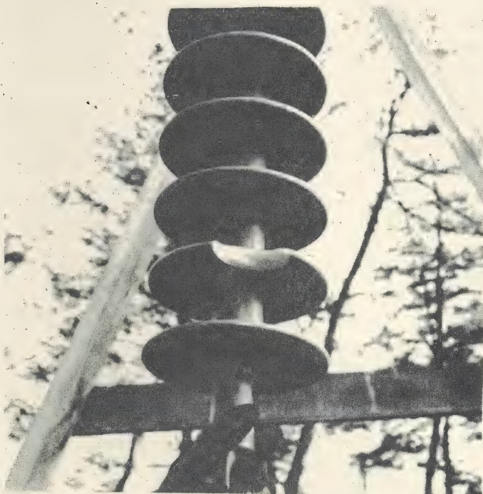
FIG. 3 --- .22 CALIBRE RIFLE DAMAGE
