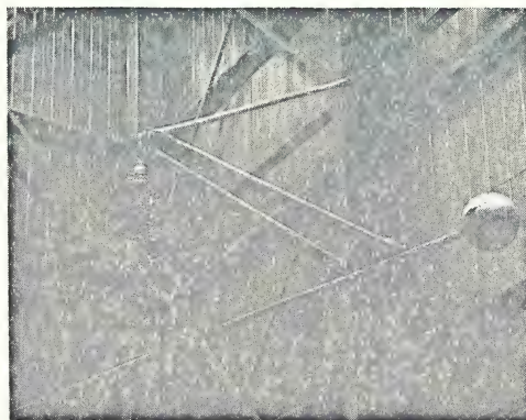
Fig. 1. Six-foot ECA crossarm with five suspension insulators. Electrical characteristics: 60-Hz flashover—714 kV dry, 431 kV wet. Impulse flashover—1174 kV positive, 1255 kV negative.
