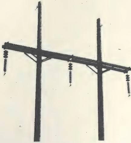
1. Polymer Insulators - Baltimore Gas & Elec. Co. 110 Kv
