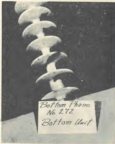
Fig. 1. Insulator returned from Jersey Central Power and Light Co. damaged by leakage currents.
