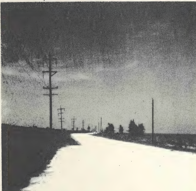
3. Polymer Insulators - Florida Power & Light Co. 69 Kv
