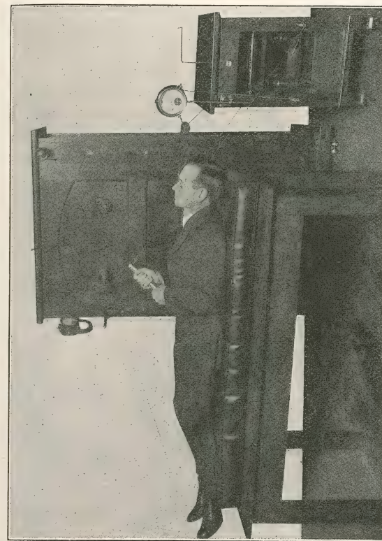
Fig. 18—Interrupterless Transformer, with Resonator Employed in Giving Auto-condensation.
