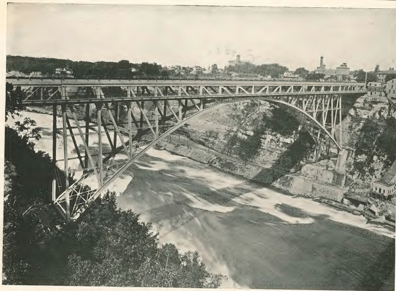
THE LOWER STEEL ARCH BRIDGE — Here is offered a glimpse of the little trolley line which skirts the bottom of the gorge from Niagara Falls to Lewiston.
