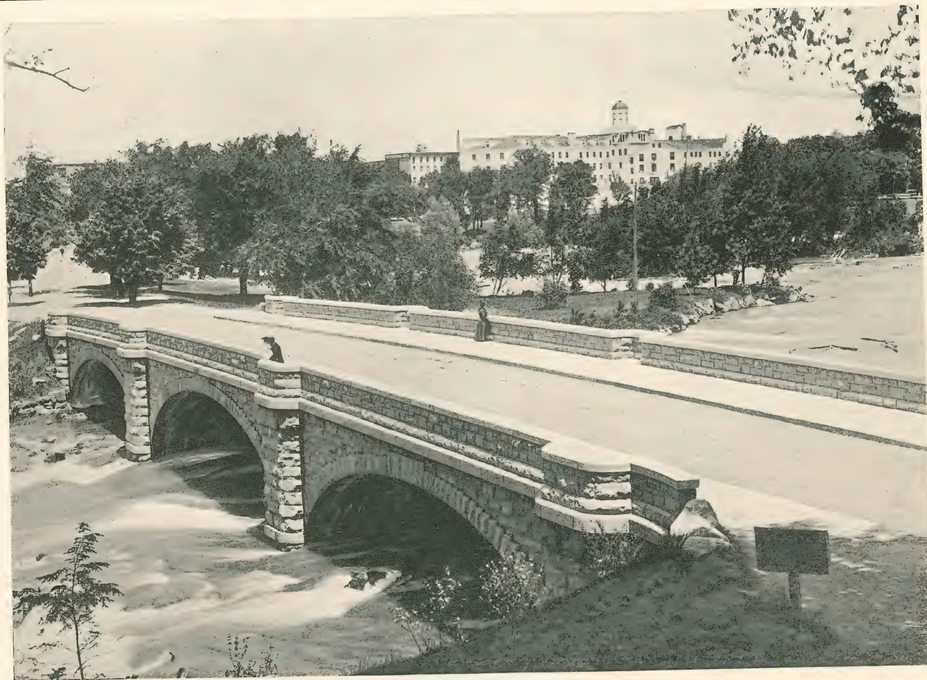
GOAT ISLAND BRIDGE — Showing Cataract House and International Hotel.
