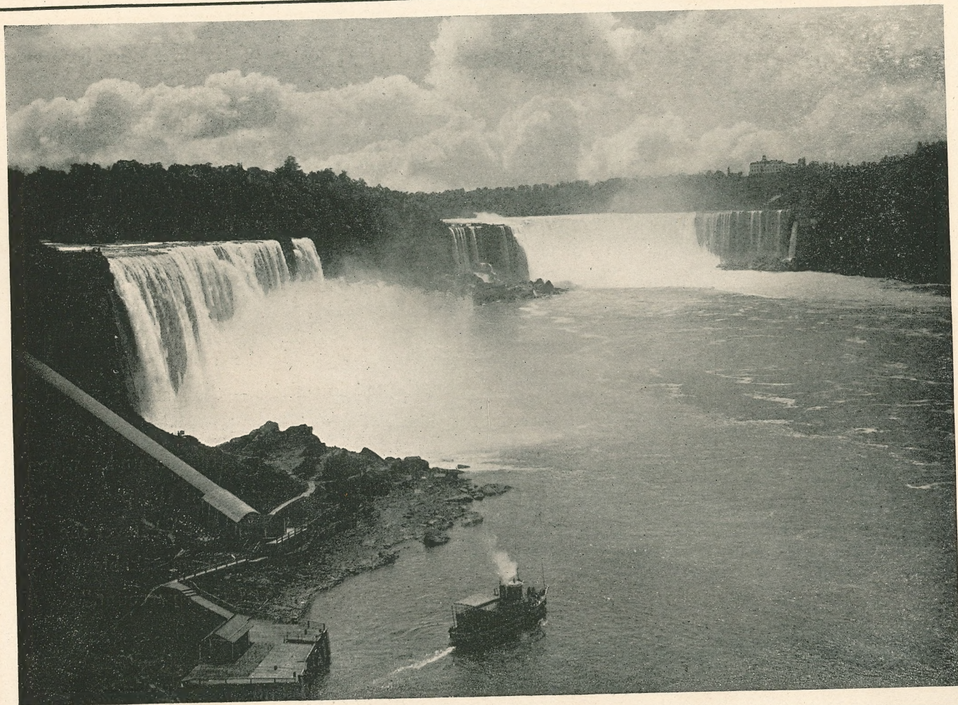
GENERAL VIEW OF NIAGARA FALLS—Showing the American Fall at the left—the Canadian or Horseshoe Fall on the right, also the inclined plane which carries people down the steep side of the gorge to the steamboat landing.
