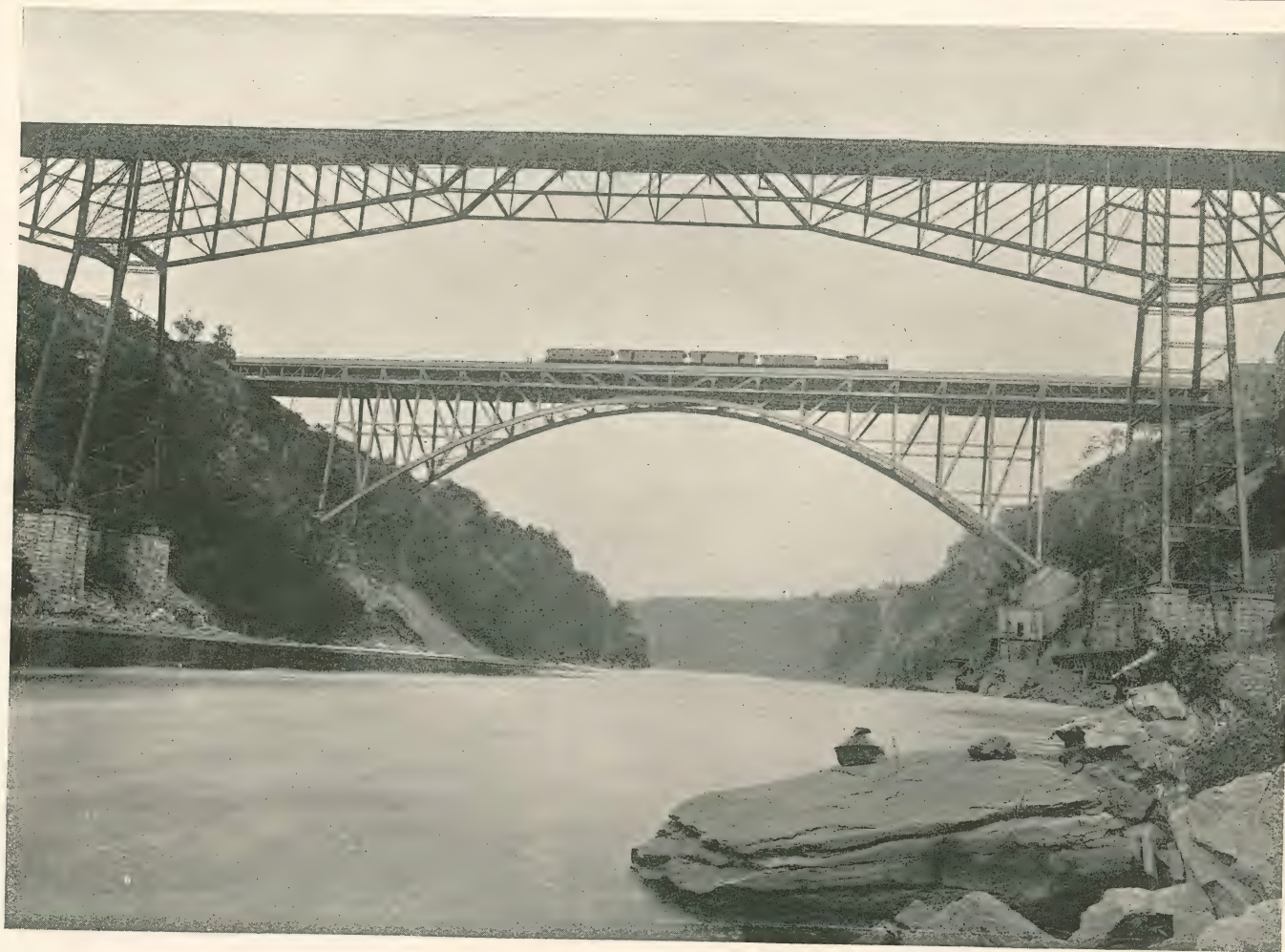
GRAND TRUNK STEEL ARCH AND MICHIGAN CENTRAL CANTILEVER BRIDGES — In the foreground is the double-track cantilever bridge of the Michigan Central Railroad, built 1883. It is 900 feet long. The towers which support it rise 135 feet above their piers. The Steel Arch Bridge beyond was built in 1897, for the use of the Grand Trunk Railway.
