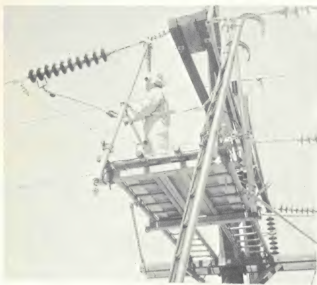
Figure IV-13. Lineman on Bare-hand Platform Wearing Conducting Suit Making a Test of Insulation Using the Live Line Insulator Tester.
