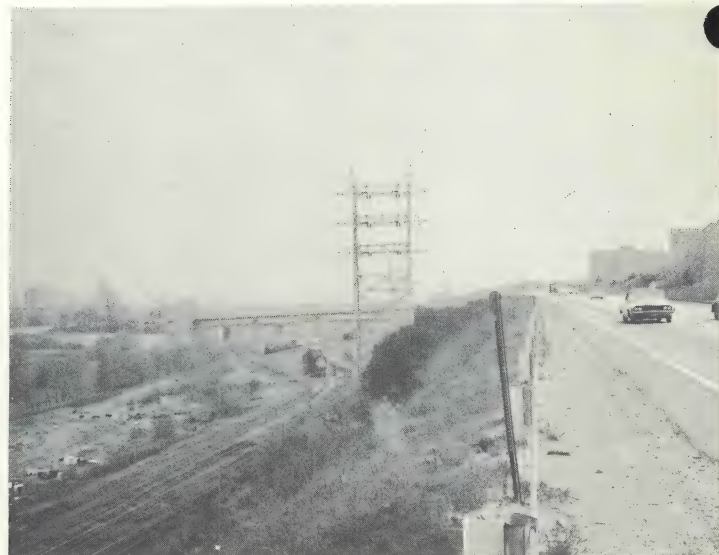
Figure IV-4. Four-Circuit 69KV Line Located on Bank Between a Railroad and an Expressway
