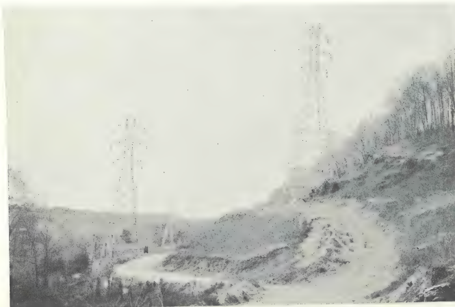
Figure IV-3. Typical 69KV Lattice Steel Tower Line Located on Hilly R/W.
