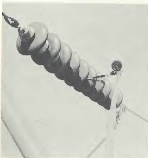
Figure IV-11. Checking Insulator Condition Using the Live Line Insulator Tester.
