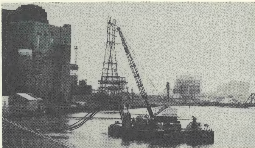
FOUR 4-IN. I.D. CONDUITS feed into the injector to be buried 8-ft under "bottom"
