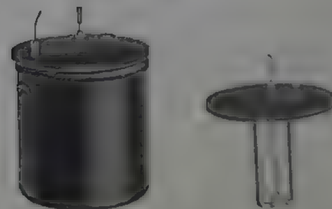
Electrolytic Interrupter.
