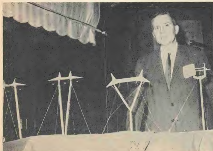
NEW GUYED-Y TOWER for 500-kv lines (second from right) is compared with more conventional guyed structures by V. F. Crowley, Shawinigan Engineering Co.
