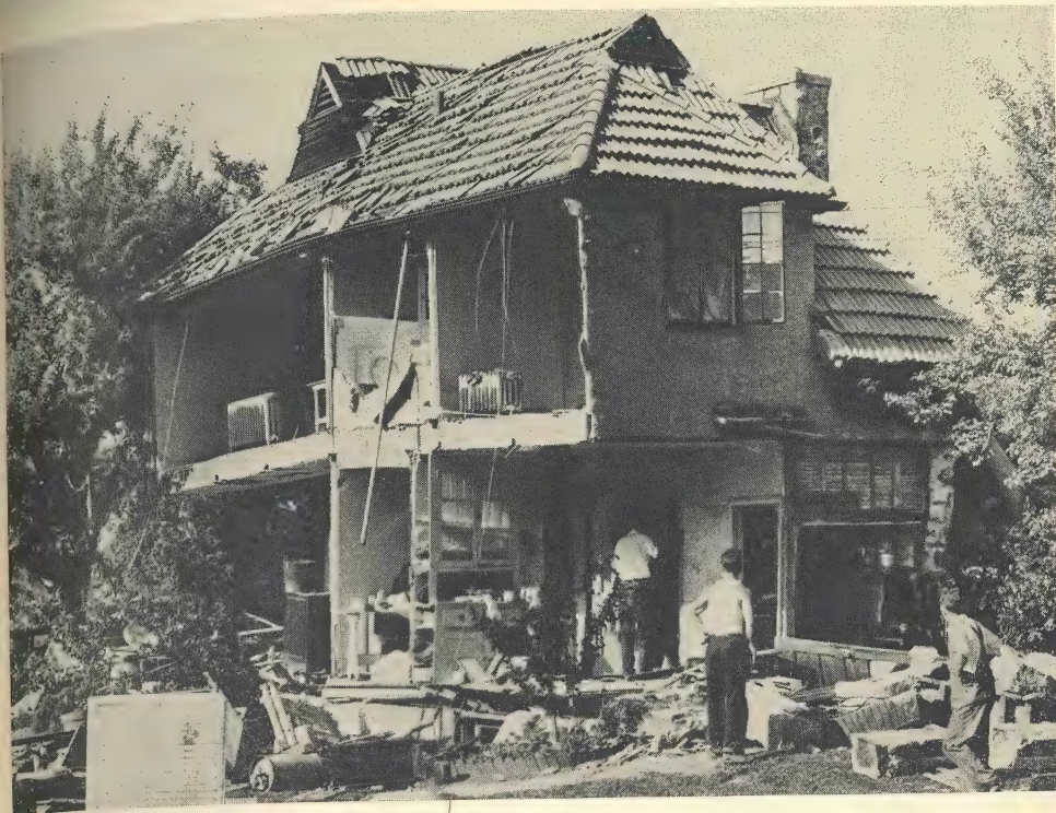
The home of Julius Saxton, White Plains, New York, following a lightning stroke during a storm on June 21, 1936.
