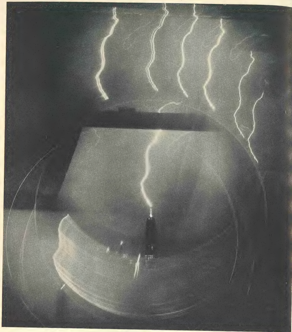
Stroke No. 16, taken in August, 1937. Still-lens photograph is in center. Rotating-lens record begins at lower left with an upward stepped leader followed by continuous current as long as illumination persists. This initial continuing discharge is followed by six further discharges, each of which has a downward continuous leader.
