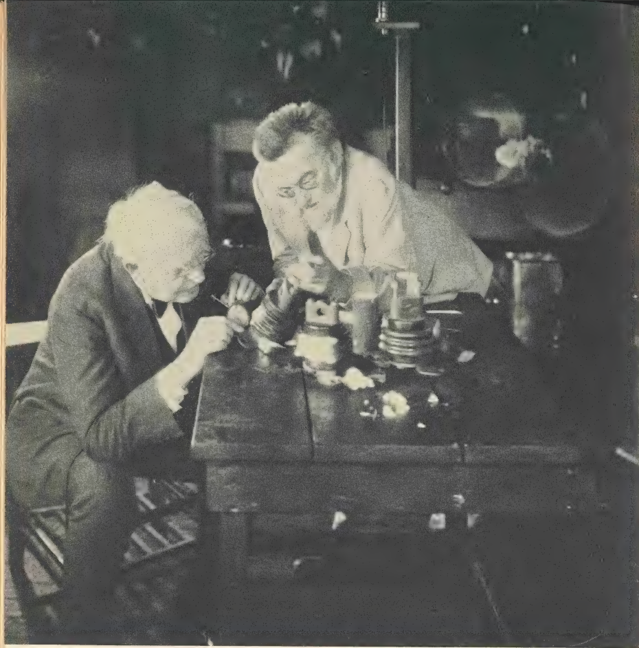
Edison and Steinmetz examining a porcelain insulator damaged by a laboratory lightning discharge.
