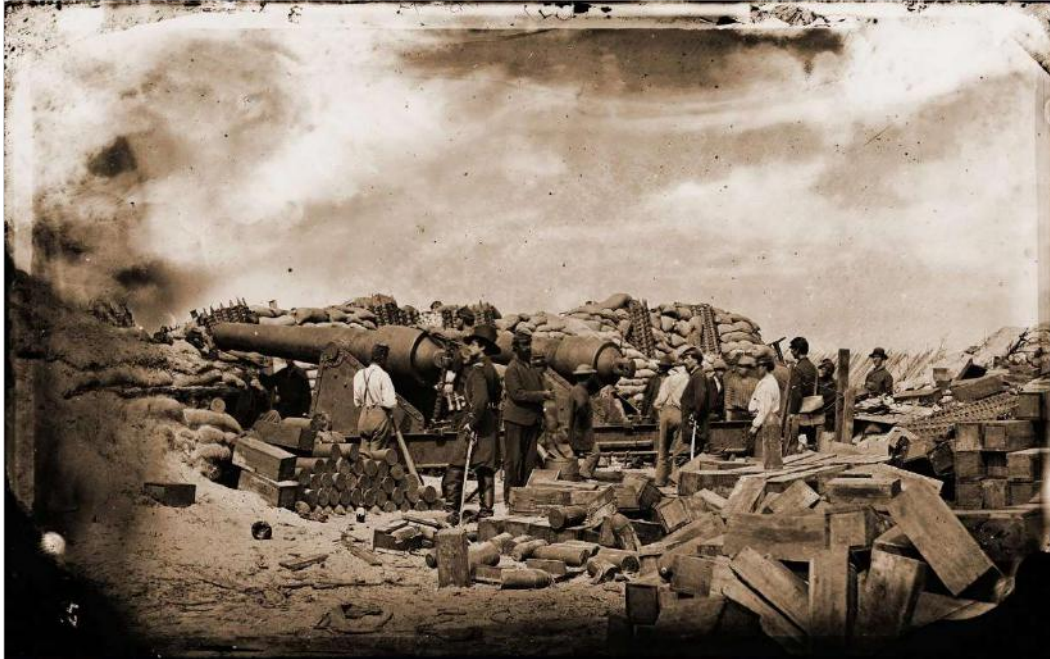
Battery Rosecrans, 2 d Parallel of Federal siege works on Morris Island, S.C., serving as a breaching battery against Fort Sumter and consisting of three 100-pounder Parrot Rifles (ca. July-August 1863)
