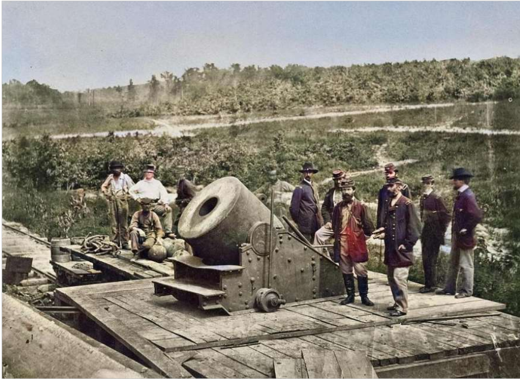
"The Dictator" mortar fired 200-lb. shells 2-½ miles from a reinforced railroad car, Petersburg, Va. (September 1, 1864)
