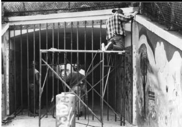
Welders close the tunnel.
