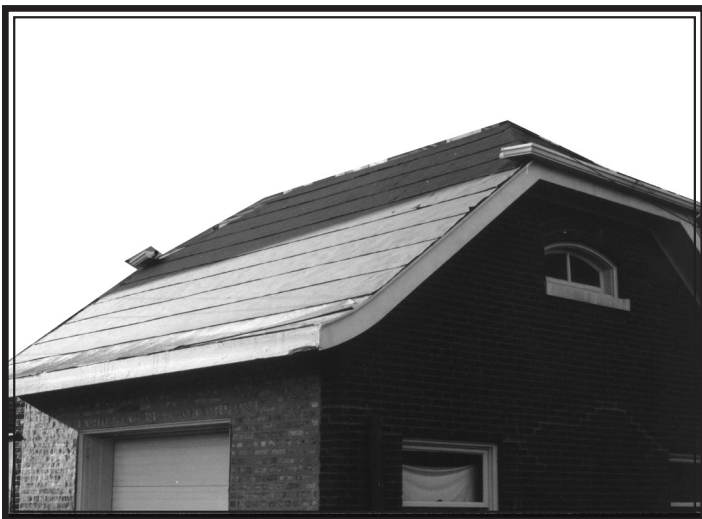
Tar paper and ice shield are installed on the coach house.
