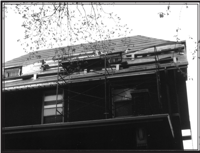
Tar paper and ice shield are installed on the wooden roof.
