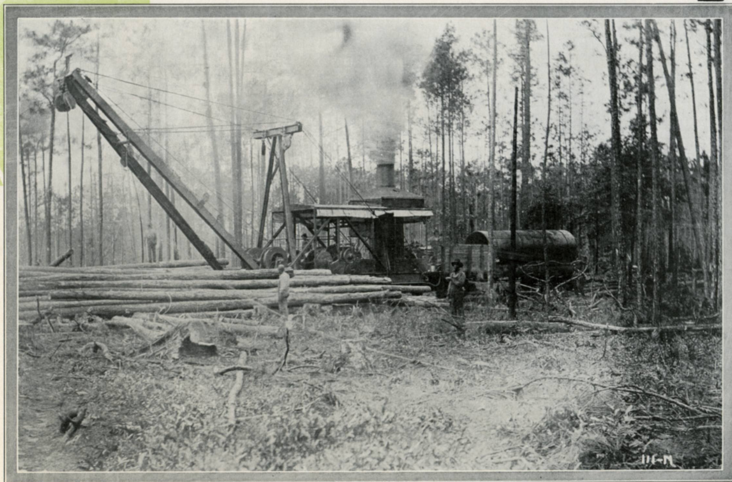
Clyde Two-Line Single End Skidder with Cable Outhaul.
