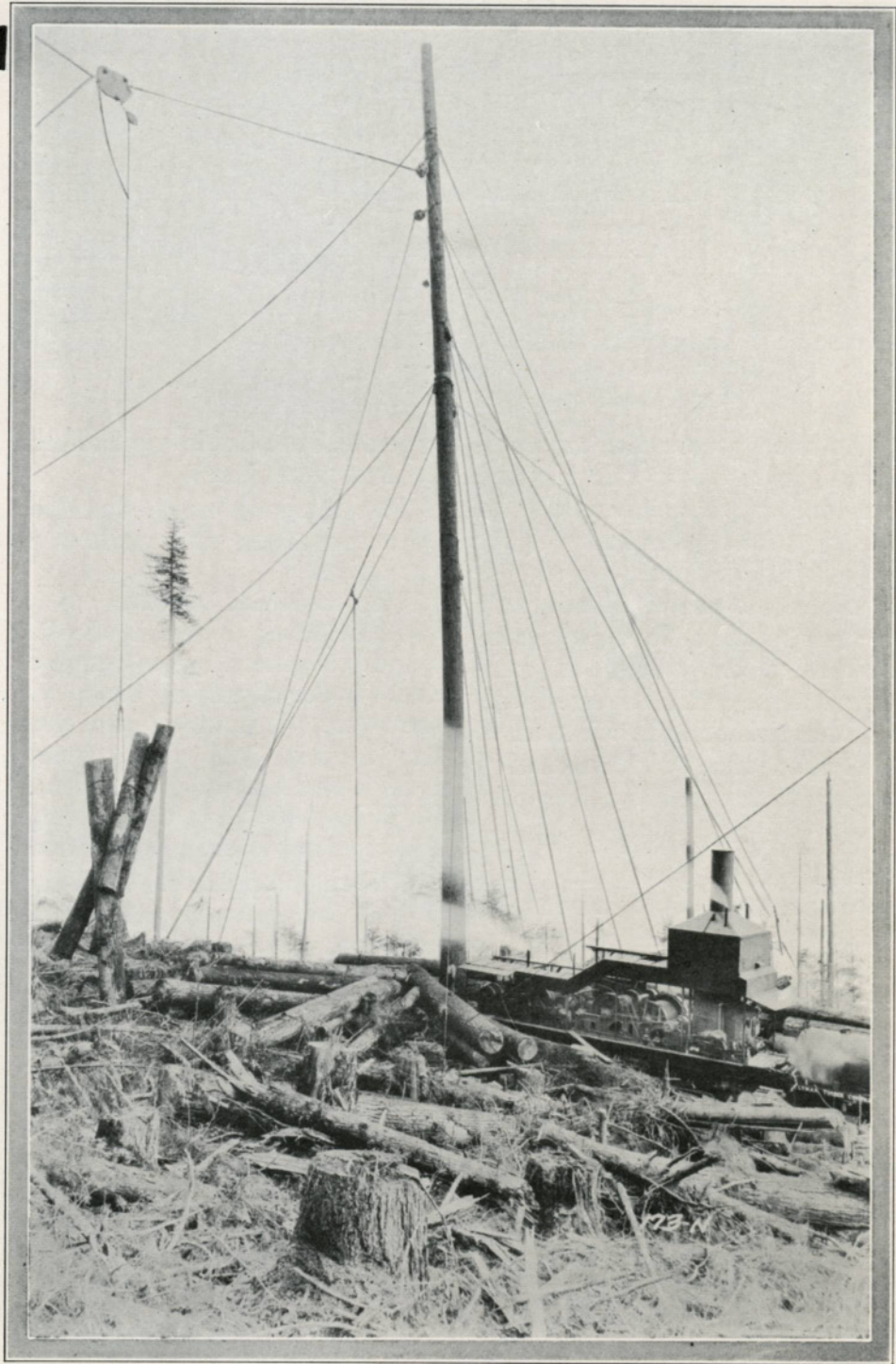
Rigging of Tree for Clyde Western Type Cableway Skidder and Loader.
