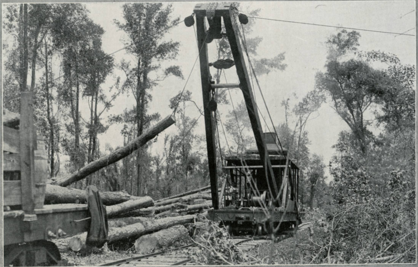
Clyde Two-Line Single End Skidder for Horse Outhaul.
