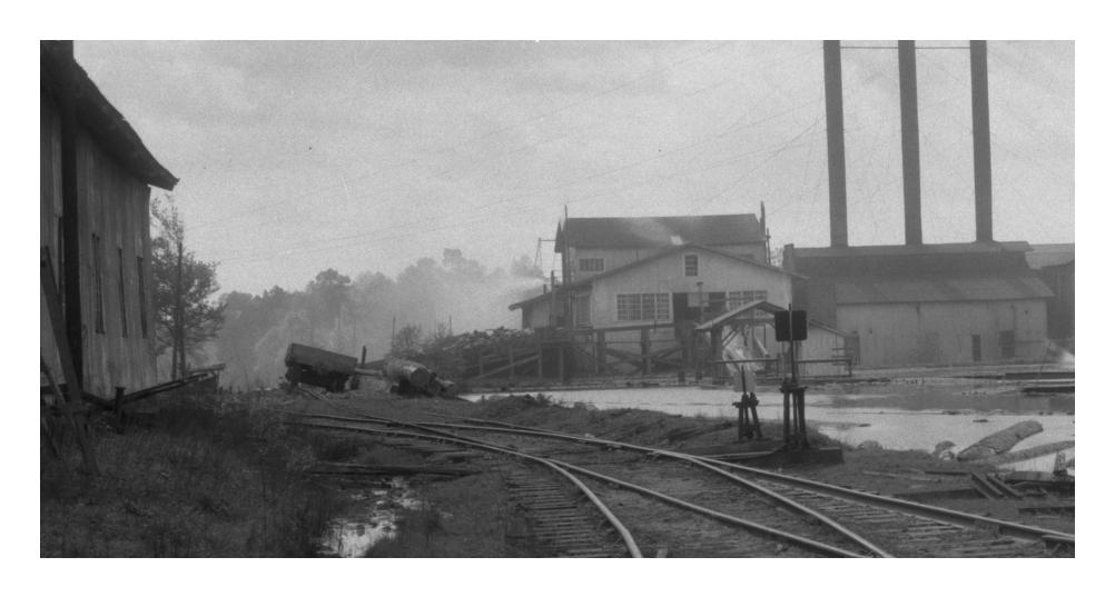
In an enlargement of the previous view, you can see the gondola perched on the end of the leaning log unloading track and the switches leading to the unloading track, as well as the connecting track leading down the hill to the M.P.
