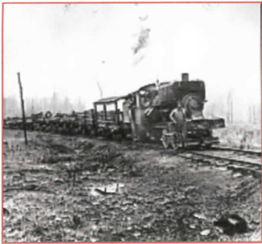
Carrier Lumber & Manufacturing Company log train on the company-owned Sardis & Delta Railroad near Sardis, Mississippi. The Heisler locomotive was one of the three major types of geared locomotives used widely in the Mississippi woods. The high firebox made the Heisler a favorite of Mississippi Delta hardwood loggers because it could wade through frequent flood waters that covered the tracks. Photo from Dr. Gilbert H. Hoffman. Courtesy, Collection of Tony Howe-Gilbert Hoffman-David Price.
