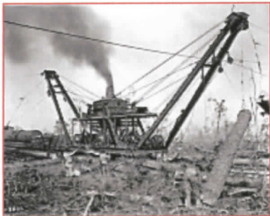
J. J. Newman's Clyde four-line skidder at work in Jefferson Davis County. J. J. Newman had huge sawmills at Hattiesburg and Sumrall. Sumrall was founded as a sawmill town for J. J. Newman. The Clyde skidder could gather fallen timber from as far as 1,000 feet from either side of the rail logging spur. Logs were stacked next to the spur and later loaded on log trains. Photo from S. E. Moreton, Jr. Courtesy, Collection of Tony Howe-Gilbert Hoffman-David Price. Larger view
