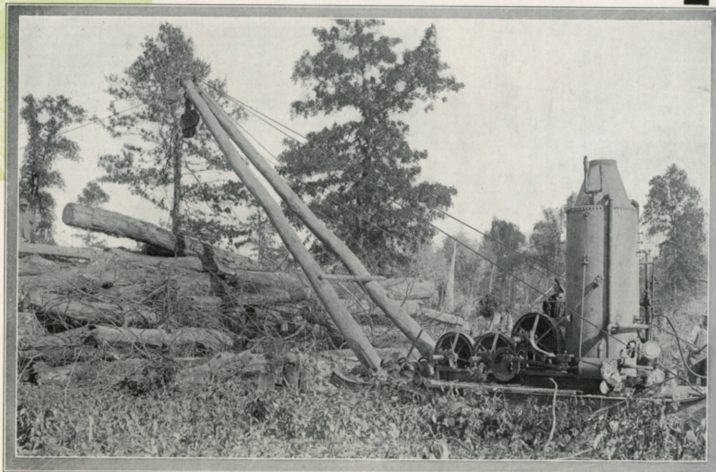
Clyde "Rapid" Ground Skidder for Operating Two Skidding Lines.
