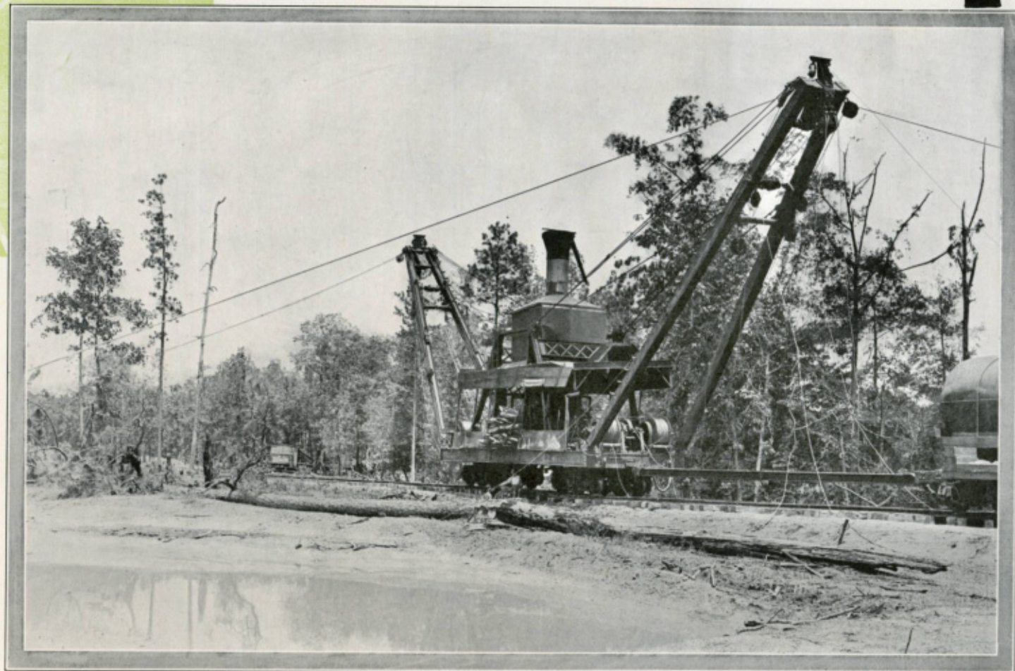
Clyde Four-Line Skidder with Cable Outhaul.
