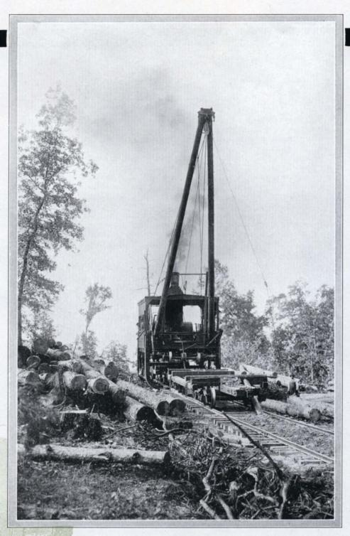
McGiffert Loader with Rigid Boom, trucks raised and cars passing through.
