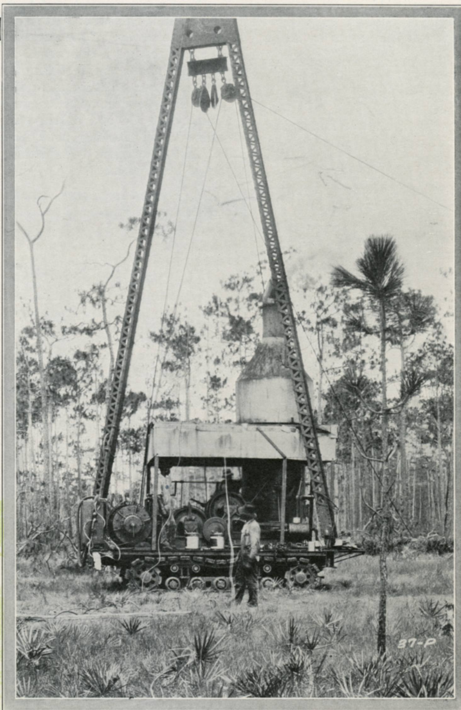
Clyde Traction Skidder for Operating Two Skidding Lines with Horse Outhaul or One Skidding Line with Cable Out- haul.
