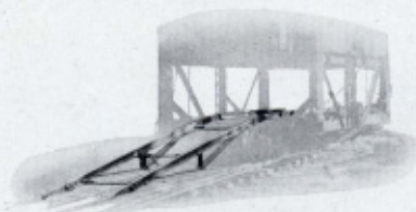
Incline track on Clyde Decker Loader lowered on track in position for passing cars through the machine.
