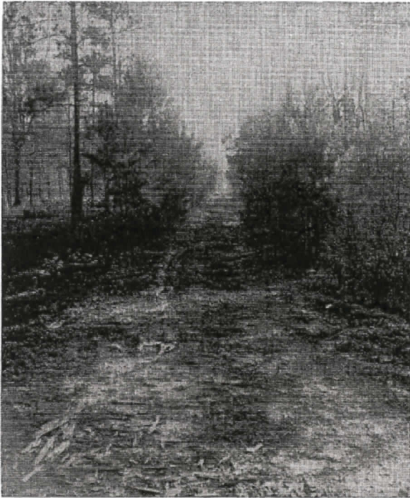
FIG. 15. Abandoned logging tram near Ward, Allen Parish, Louisiana, now used as a road for logging trucks. Many stretches of track have been improved and incorporated into the permanent road system.
