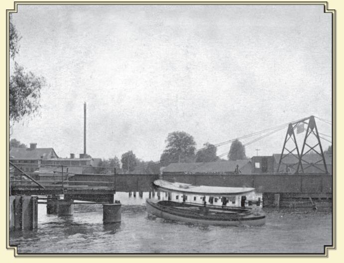
5 - SWING BRIDGE ca 1910 In 1902 a swing bridge replaced the 1870 drawbridge at that location. A keeper minded the bridge during the navigation season. In 1936 the Blue Star Highway was opened and it included a huge causeway leading to a fixed span of the type in use today.
