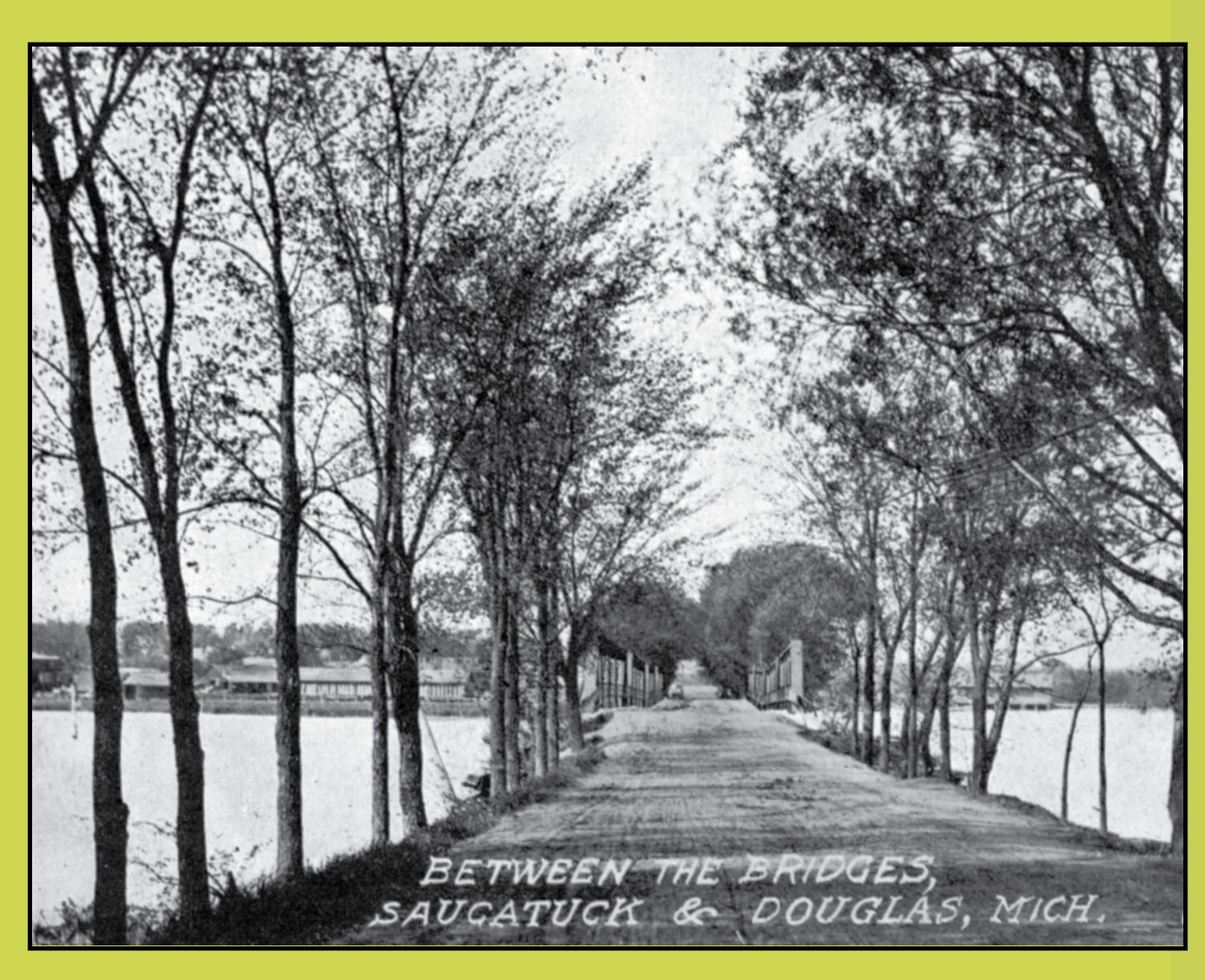
THE FIRST BRIDGE between Saugatuck and Douglas was built in 1868, and the crossing included an approach, a long low stationary bridge (pictured here) which continued across an island in midstream and then a draw section (later replaced by a swing bridge) which opened to allow passage of boats upstream.
