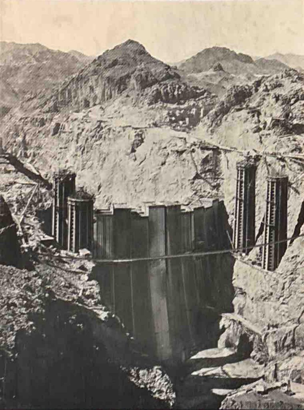
A construction view in November, 1934, of the Dam and Intake Towers. The Dam is approximately 600 feet above its base and 130 feet below its crest. Cylindrical gates in the Intake Towers will regulate the flow of water from the reservoir to the power plant.
