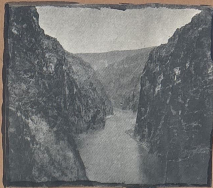
Black Canyon Boulder Damsite May, 1931
