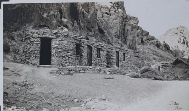
Stone Cabins erected by the C.C.C. Unit #573 - Ohio Boys.
