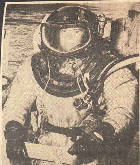
NOT IN THE OCEAN —Diving is not limited to the deep sea, as witness this Lembke Construction Co. employe ready to go down in the tailrace of the Hoover Dam powerplant on the Colorado River. The contractors, who have the job straightening the roadway structure at the Nevada wing of the powerhouse required the services of a professional diver last week when they were ready to pour underwater concrete. Two divers went down to take measurements, and later sealed off the bottom of underwater forms.
